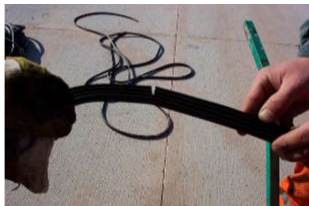
Figure 11: Joint profile installation equipment for transverse joints of a highway in Austria (ÖAT 2;, 2020)
