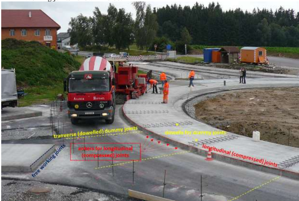
Figure 37: Different types of joints using the example of a roundabout in Upper Austria (Hrapović 2, 2020, S. 259) (supplemented by author)
