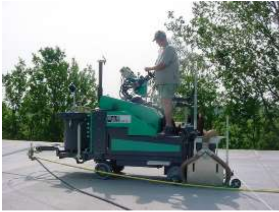
Figure 5: left: cutting the concrete ceiling in a slot width of 2.0 to 3.5 mm (Alte-Teigeler)
