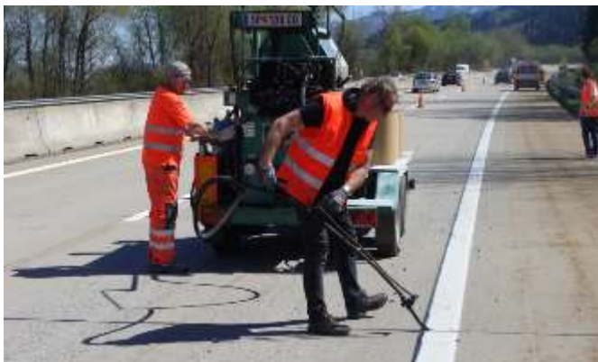
Figure 14: Grouting of joints in the hot grouting process (ÖAT 3,; 2020)
