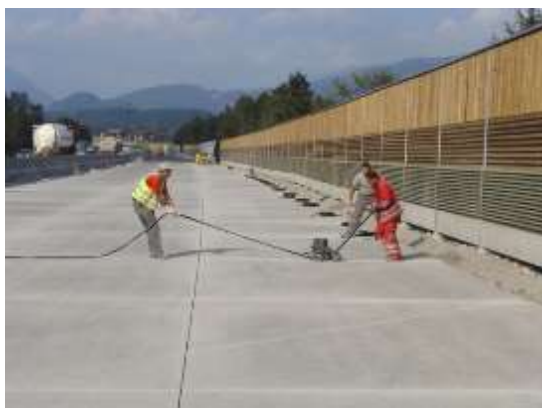
Figure 11: Joint profile installation equipment for transverse joints of a highway in Austria (ÖAT 2;, 2020)
