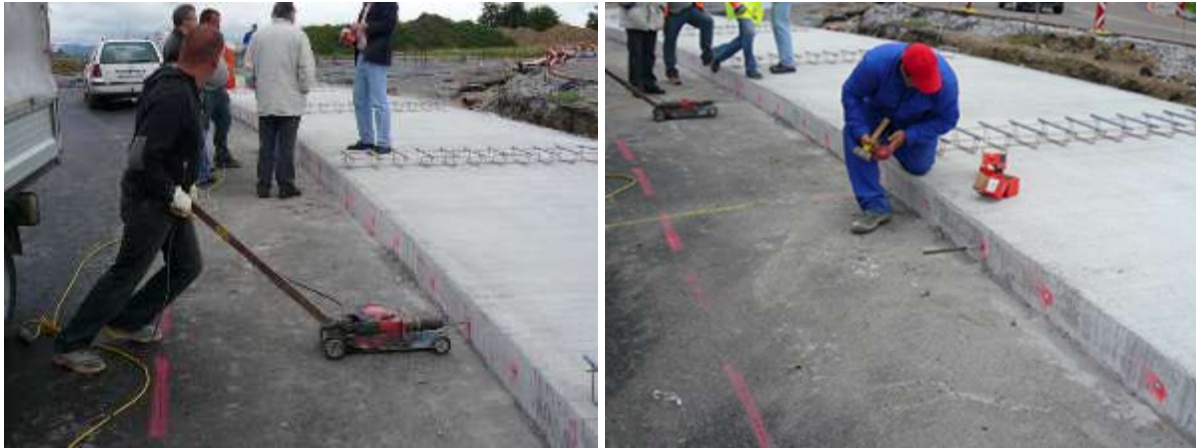
Figure 35: Ingenious system for drilling holes for hammer-in anchors (Hrapović 2, 2020, S. 254)
