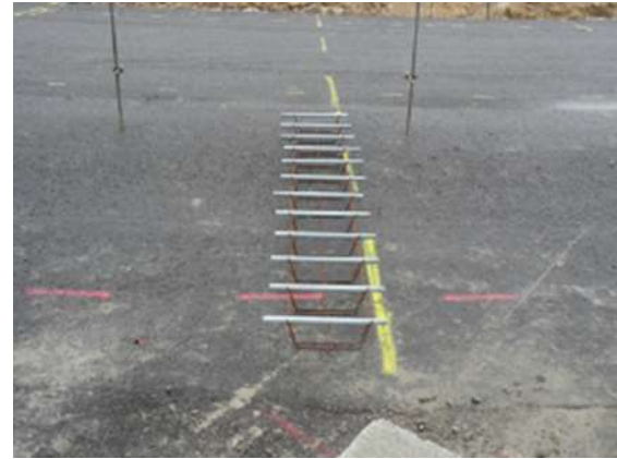
Figure 24: Dowels installed for the transverse joints of a roundabout in Upper Austria (Hrapović 2, 2020, S. 248)
