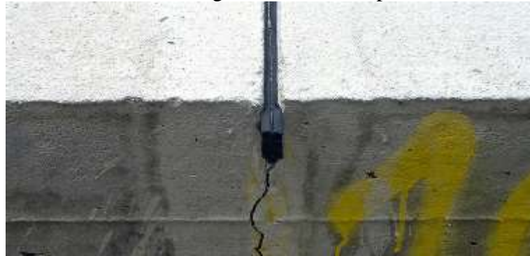
Figure 10: Example of an elastic jointing material (ÖBA, 2020)
