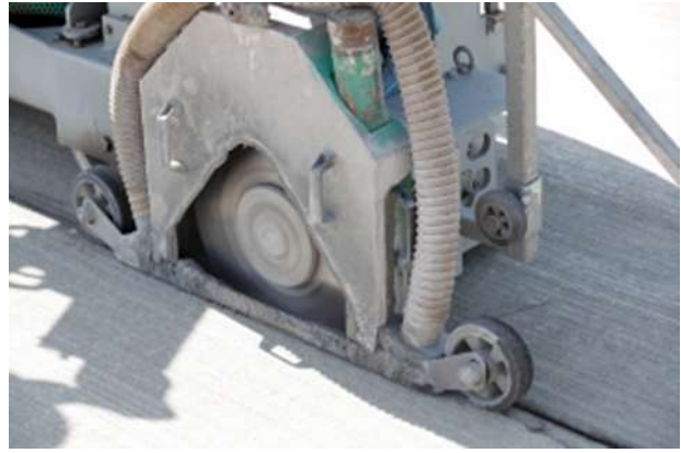
Figure 5: left: cutting the concrete ceiling in a slot width of 2.0 to 3.5 mm (Alte-Teigeler)
