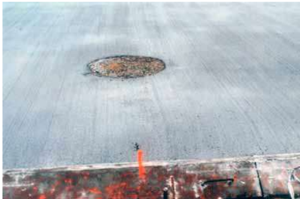
Figure 17: Example of a parting line around the manhole cover (ECPA, 2013, S. 12)
