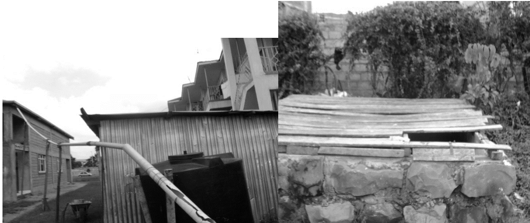
Figure 4: Improvised mechanism for harvesting rain water by a church in Embakasi; from left is the piping system followed by an underground concrete storage reservoir.
