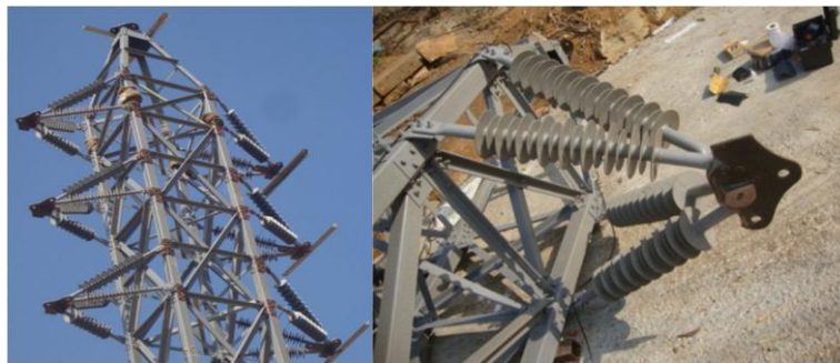
Figure 4 Composite cross arms on tower body
