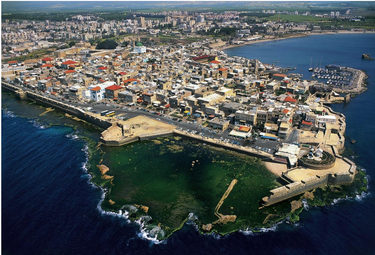
Aerial view of the Old City of Acre shows its harbor, the ancient walls and the Al-Jazzir Mosque.
