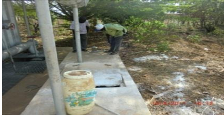
Figure 4. Inspecting Improper dosing of disinfectant (HTH) at Ibi-Wukari water treatment plant
