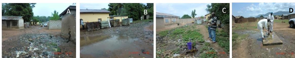
Figure 6. (A–D). Poor sanitation and hygiene practices around boreholes, hand pumps/pumping mechanisms and the location of boreholes at the downhill/down slope site
