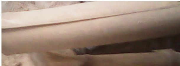
Fig., 1a: group B of bamboo culm dried in the open air exhibited cracks within 2 weeks
