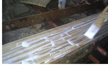
Fig., 11: Gluing of opening in the laminated bamboo
