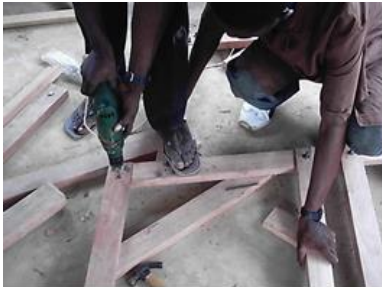
Fig., 3: Drilling holes for bolts and nuts
