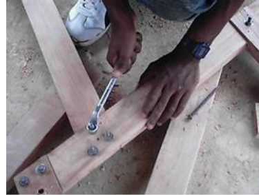
Fig., 4: Fastening with bolts and nuts
