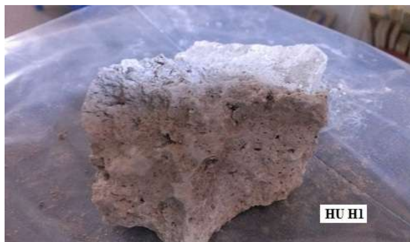
Figure 7. Mortar sample numbered HU H1 which was taken from Harran University
